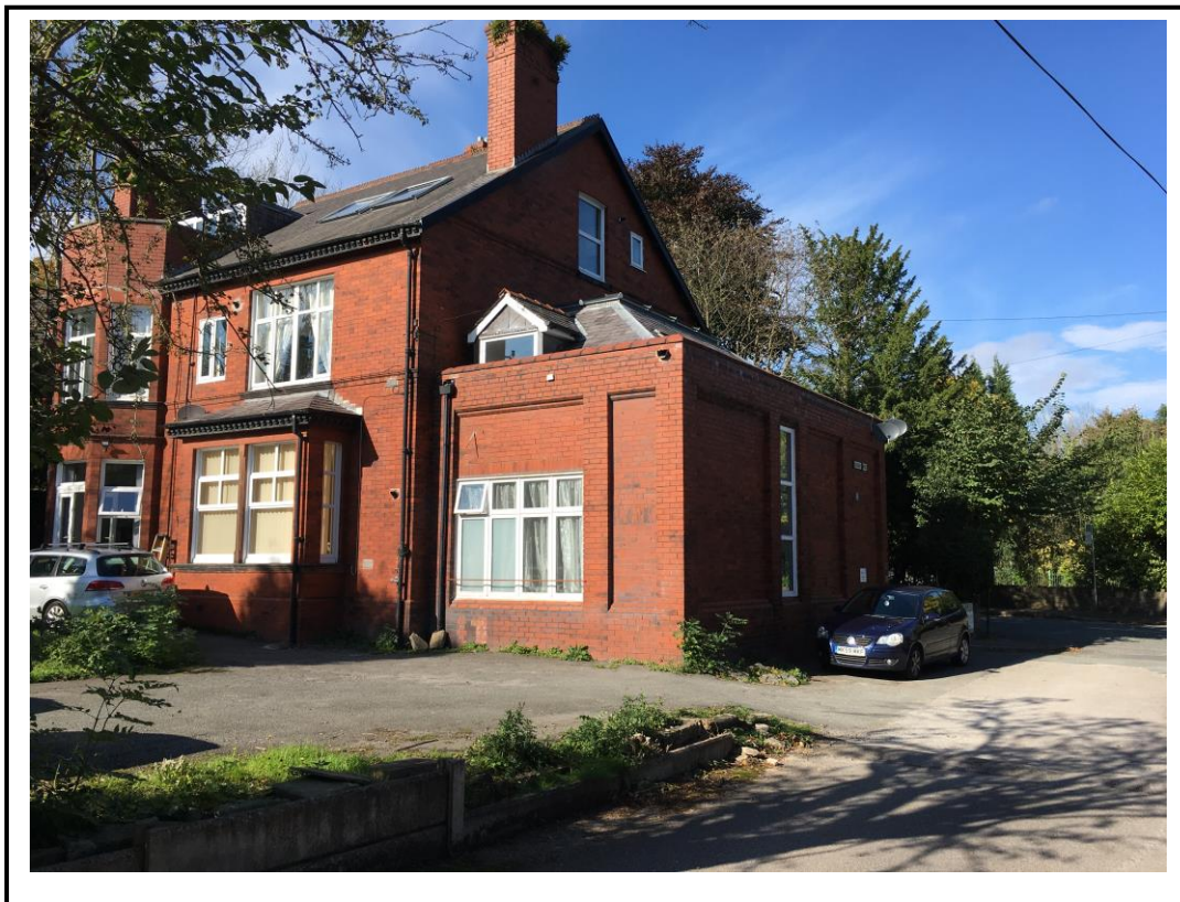
View from Rosemary Drive towards Stockport Road
